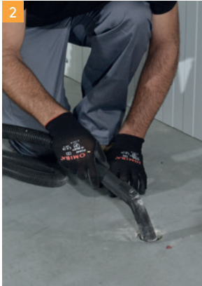
2 Ensure area is clean and free from debris.
