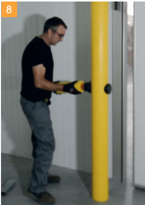
8 Fix reinforcement arm to vertical post.
