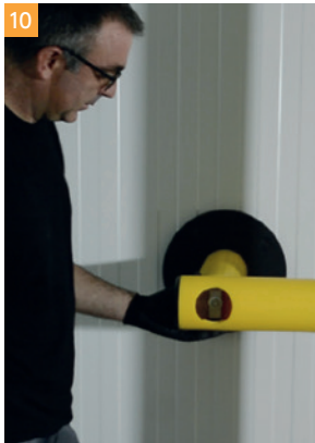
10 Assemble all reinforcement arm components and position on wall.
