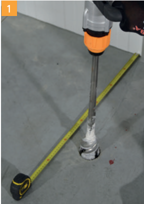
1 Measure and drill locations for anchor fixings.
